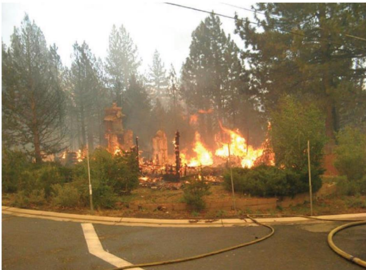
Figure 6: A destroyed home following fire spread from the Angora fire. Note the intact, unburned vegetation surrounding the structure. Murphy et al. notes that this house was ignited by wind-blown firebrands, not by surface fire spread or radiant heating (Murphy et al., 2007).
