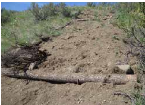
Water bars or simple log check-dams can slow erosion on steep, loose slopes.
