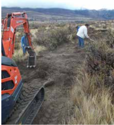
Avoid using heavy equipment like this backhoe if possible.
